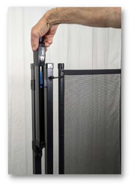
Next, Pre-drill and screw the side of the striker body to the gate frame.
