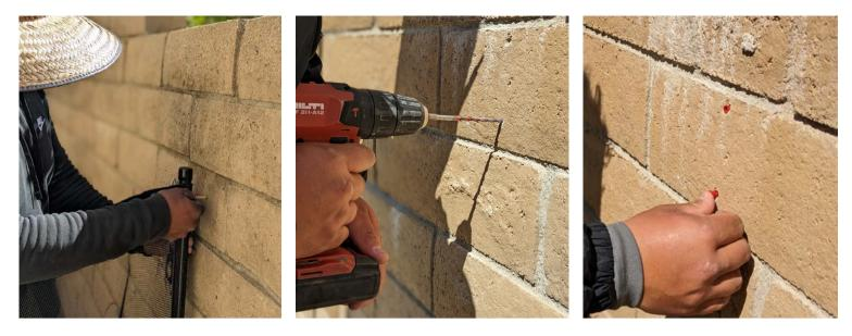
Using your torpedo level, make sure your last pole is plum (straight up and down).
