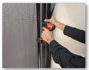
Now that your fence is connected to the gate truss and termination point, It's time to finish your end sections. We call this a Cut.
