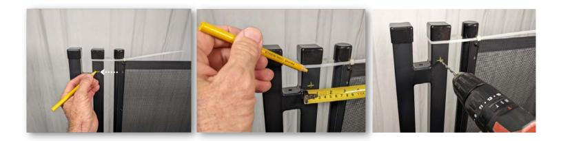
Drill the center of the truss with an 1/8" drill bit. Using the screw you removed from the pole, screw it into the truss and then remove it. This will pre-thread the hole for the section latch which you will now screw in the eye of the latch.
