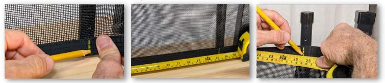
Screw only the top and bottom hole of the molding back onto the mesh at your marks. Then screw the molding and mesh to the top and bottom attaching it to the pole. Don't cut the mesh or screw the rest of the molding down yet. This will be done later.
