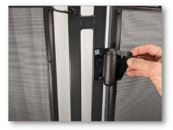
Insert a flathead screwdriver into the slot on the top of the hinge. Before you turn the screwdriver, you will need to push down to disengage the teeth holding the spring tension. **Note that when you push down, you will feel the spring suddenly try to unwind.** Do not let it unwind. Instead, you should add one notch counter clockwise and then allow the adjustment to align with the teeth and come back up.
