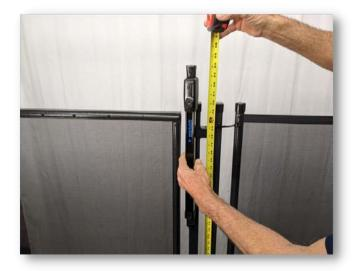
The latch location will be where the top of the pull nob is at 54" per ASTM standards
