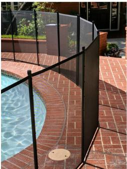
Pull the bottom loose mesh snug across the loose pole and mark the bottom border at the middle of the loose pole. Measure from the middle of your last pole to the mark you made on the border Transfer that measurement to the top border and mark it.
