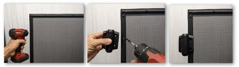
Using the black screws included with your gate latch kit, screw the hinge into the existing hole on the frame. Then, using your 5/32" drill bit, pre-drill the remaining hole and then screw it to the frame.
