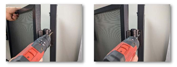
Now, slide the latch mounting brackets onto the latch. One bracket towards the top of the latch and one on the bottom.
