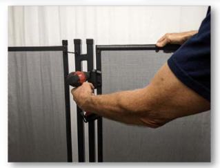
Lining up the top of the gate frame to the top border of the mesh, pre-drill the top hole and then screw it into place using the black screws. Now repeat this on the on all three remaining holes.
